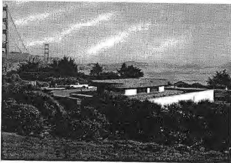
Comfort Station as seen from the sidewalk along the toll plaza.
