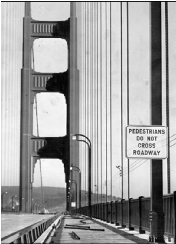
Figure 2. Photographs of sidewalk, railing, light standards and roadway. At left, just days before the bridge opened in May 1937, with original light fixtures. (San Francisco History Center, San Francisco Public Library) At right, showing replaced light fixtures, by photographer Jet Lowe, 1984. (HAER CA-31, www.loc.gov ). See Photograph 6, below for a view of the new public safety railing.
