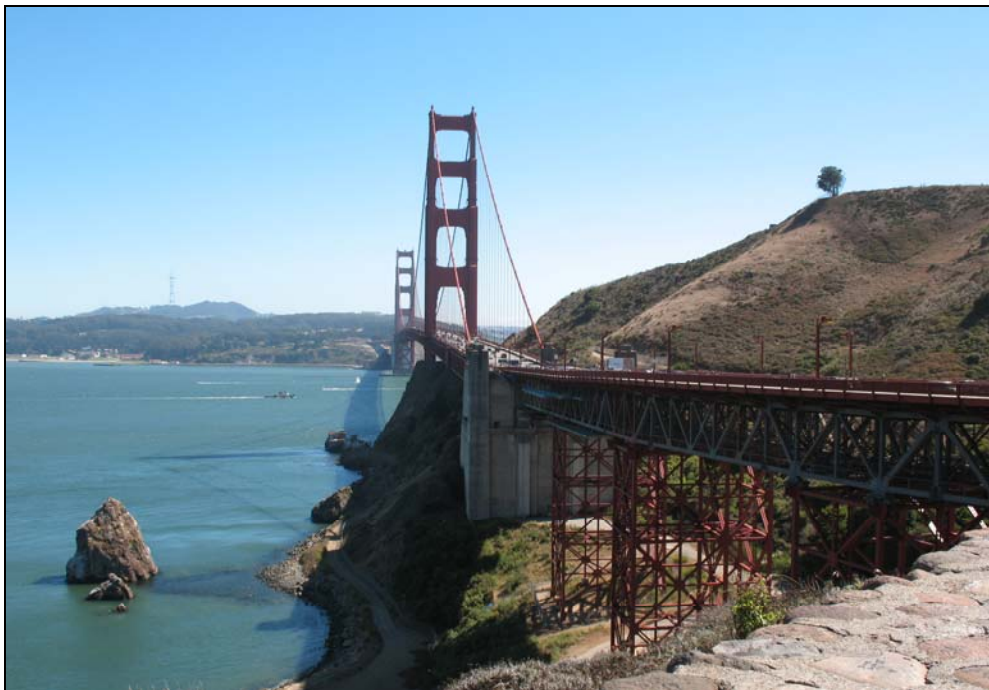
Photograph 4. View of North Viaduct from Vista Point, camera facing south. [Source: MacDonald Architects]
