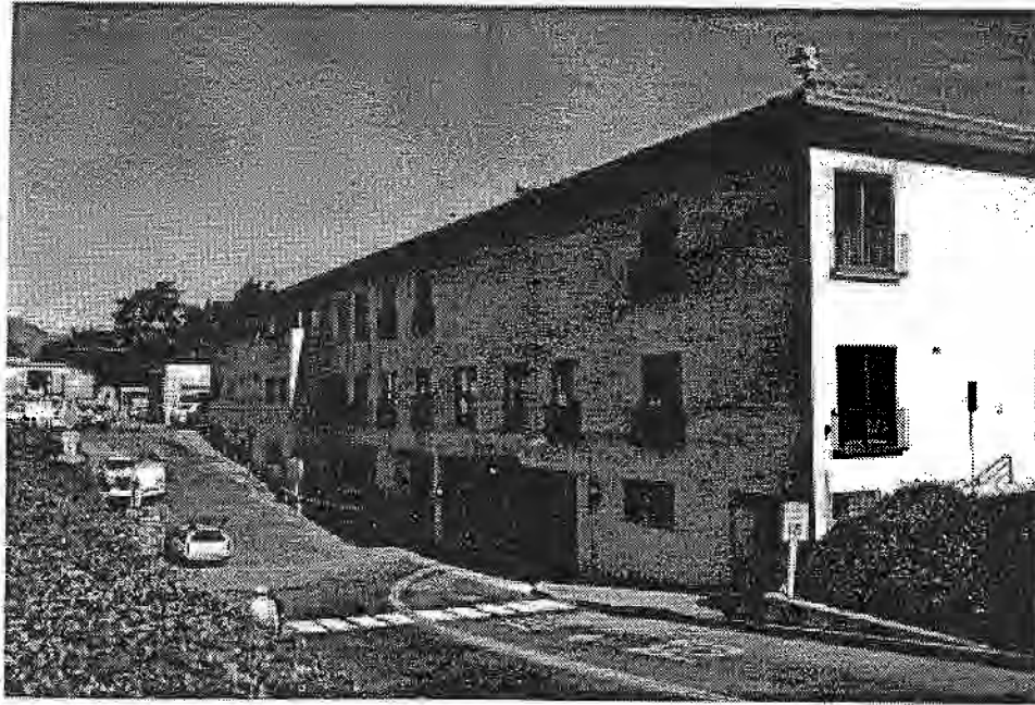
Back side (west) of Administration Building (1993)
