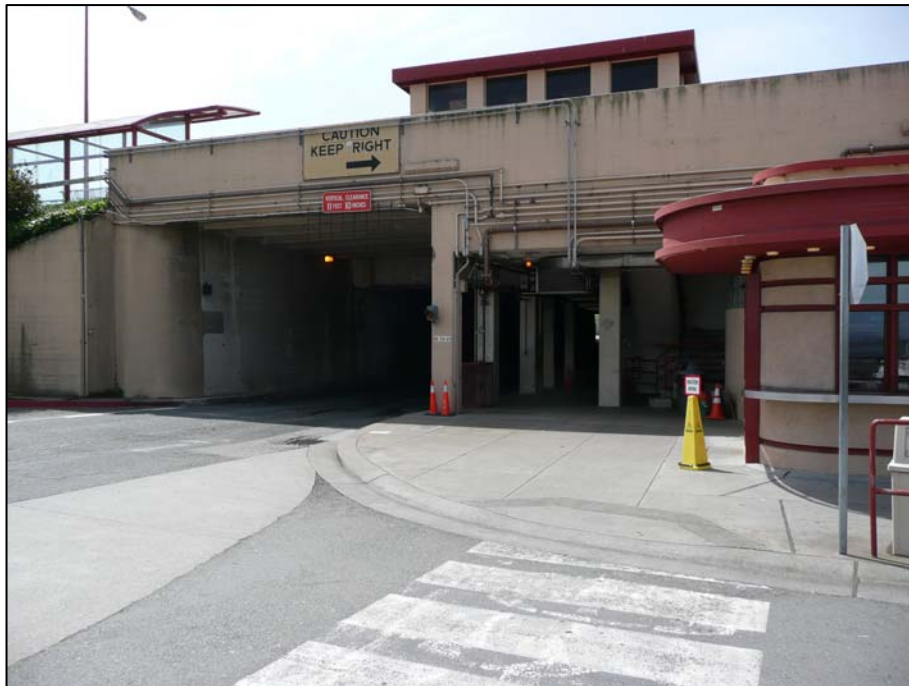
Photograph 11. East side of Toll Plaza Undercrossing (34 0069), view southwest, April 2008. [Source: JRP Historical Consulting, LLC]
