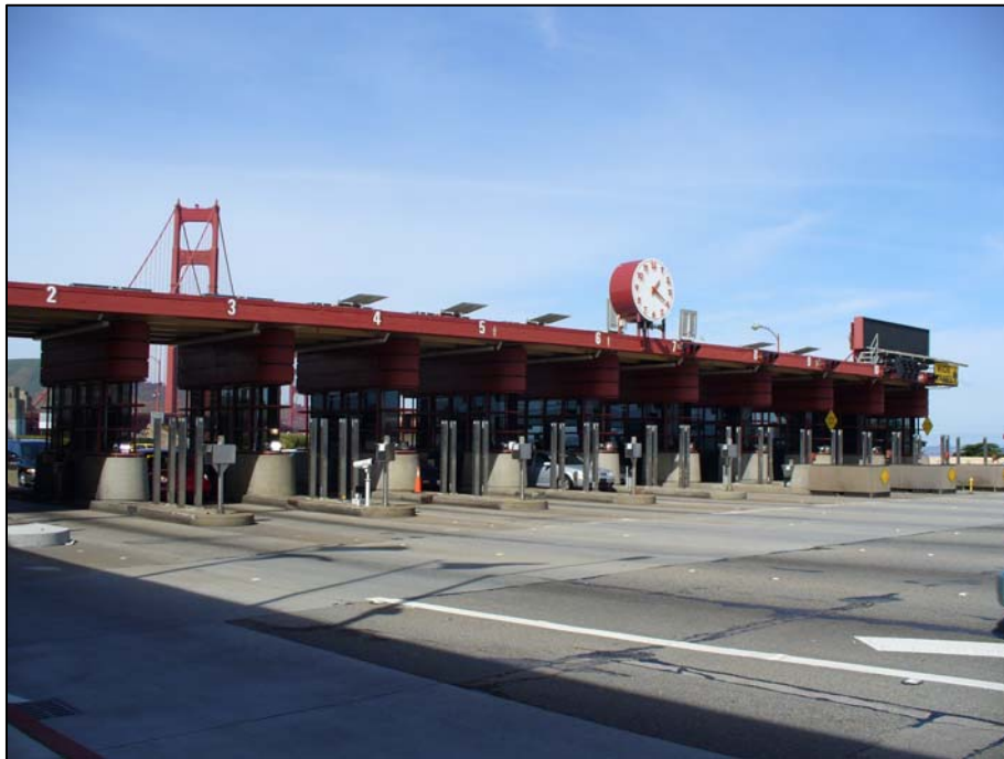
Photograph 8. Toll booths and canopy, camera facing northeast, March 2007. [Source: JRP Historical Consulting, LLC]
