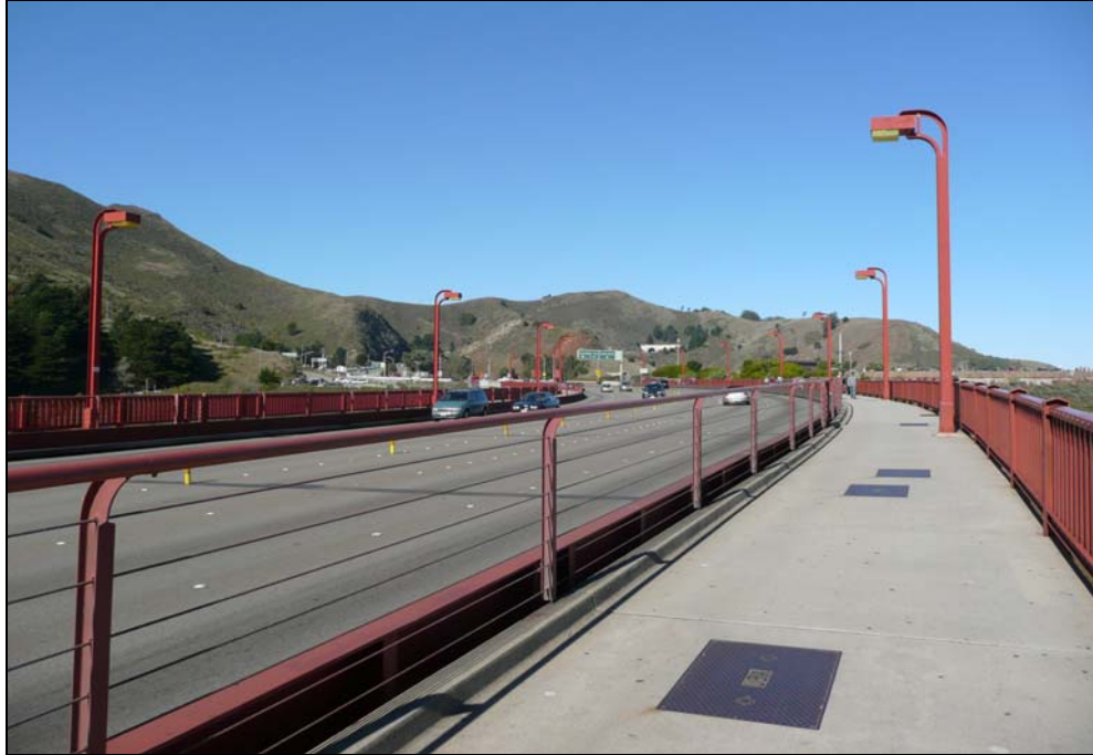
Photograph 6. View of north viaduct, showing safety railing, camera facing north, November 2007. [Source: JRP Historical Consulting, LLC]
