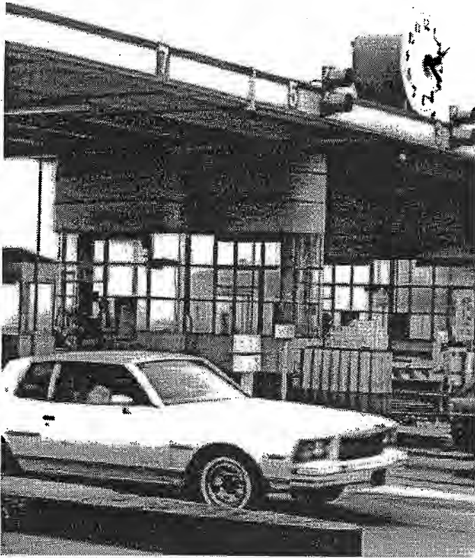
Original Toll Booths by Irving Morrow 12
