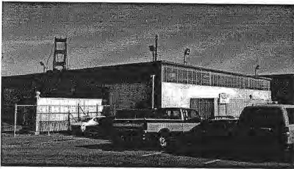
South-west corner of Maintenance Building. Note the container set in the garage door opening, and another one against the south facade.
