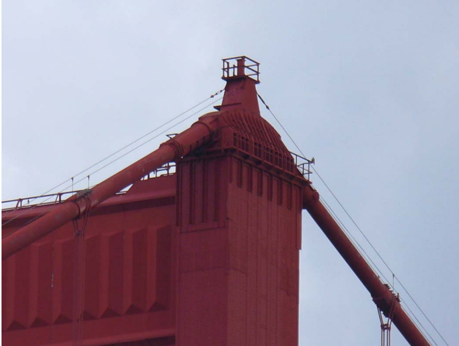
Photo B11. View of north tower of Golden Gate Bridge from survey Station 4 – Battery Spencer; looking south; February 18, 2009. Note peregrine falcon on top of railing center right.
