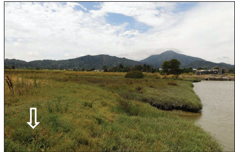
View facing west of breach area for proposed tidal connection of Project Site to northern drainage channel. Arrow indicates approximate location of tidal channel and tidal marsh for proposed project.
