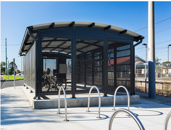
This long term, secure bike storage system was identified as a useful precedent for the Transit Center.
