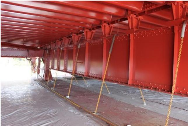
As of this writing, the South Approach Viaduct (SAV) restoration, is 90% complete. In FY 21/22, Golden Gate Bridge staff continued sandblasting, steel repairs, and repainting operations, using 218 tons of blasting abrasive and 3,195 gallons of paint and primer.
