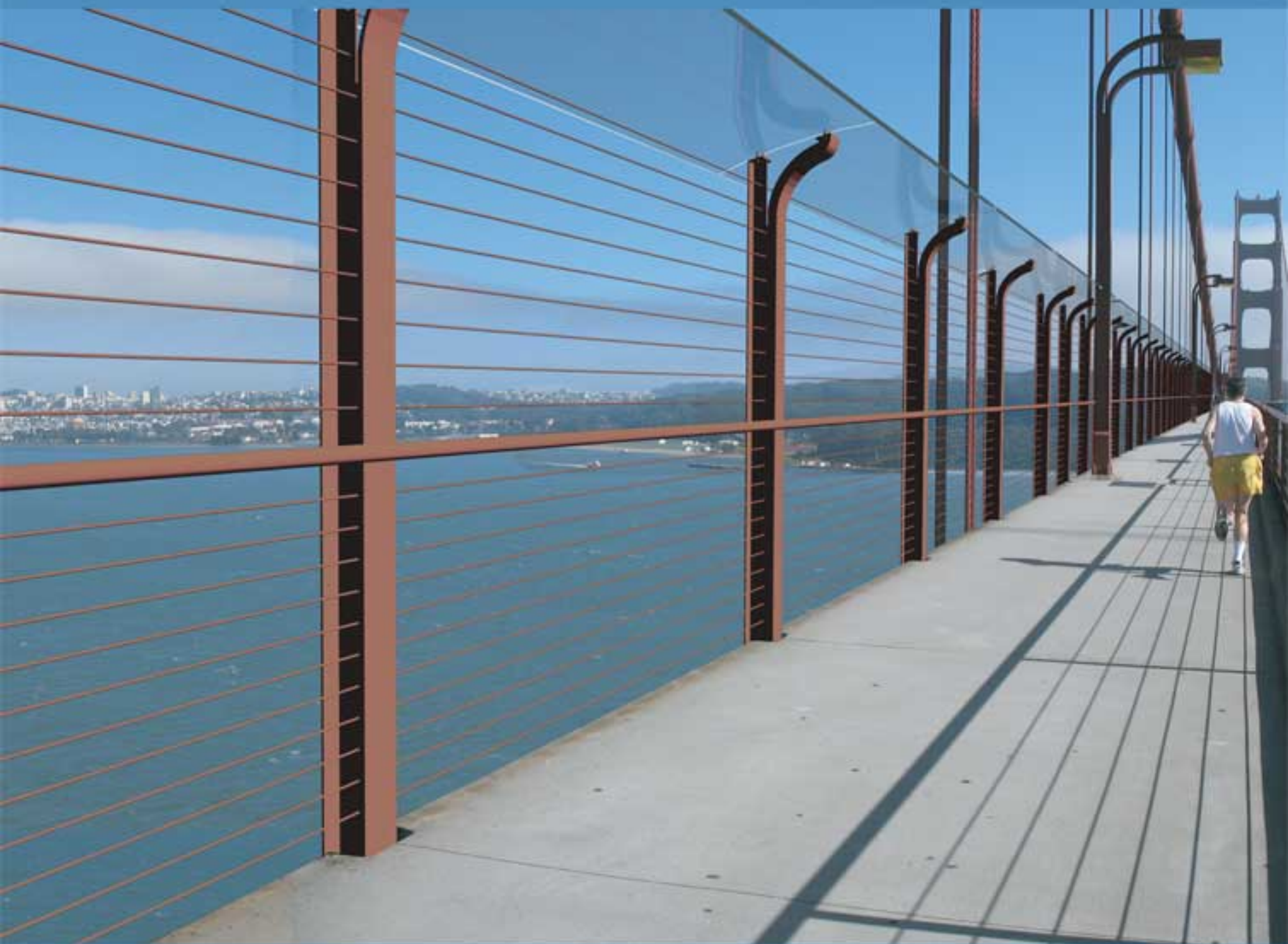
Alternative 2B - Replaces 4-foot handrail with 10-foot-tall horizontal system, with winglet Sidewalk View South
