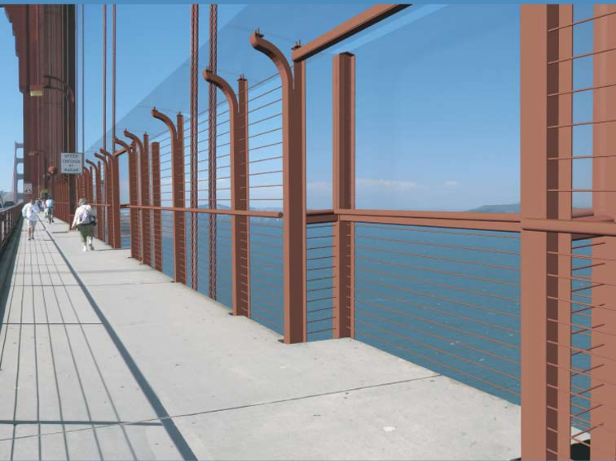
Alternative 2B - Replaces 4-foot handrail with 10-foot-tall horizontal system, with winglet Sidewalk View North
