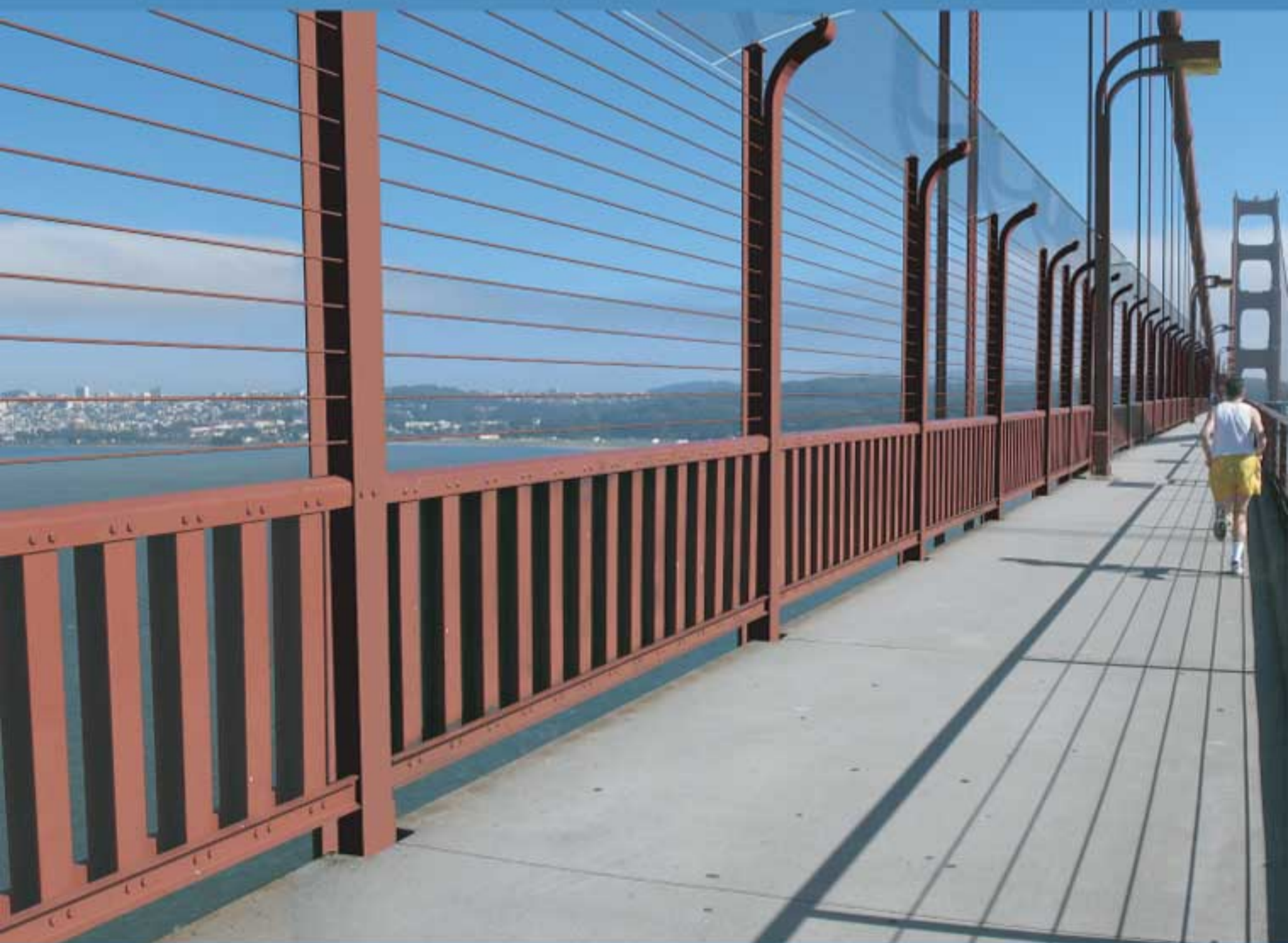
Alternative 1B - Adds 8-foot-tall horizontal system to 4-foot handrail, with winglet on top Sidewalk View South
