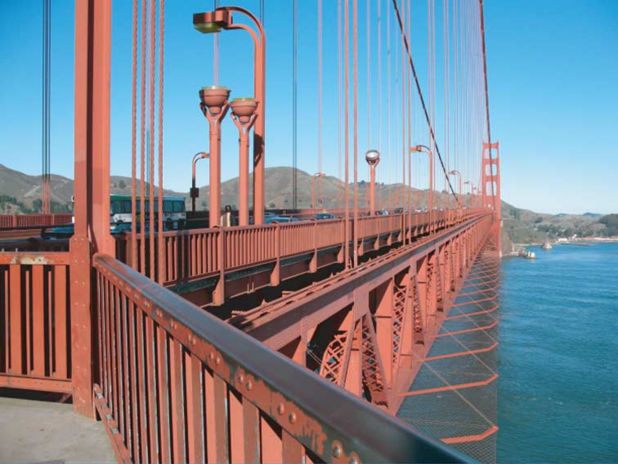
Alternative 3 - Add horizontal net system, 20 feet below and extending 20 feet out View North at Tower
